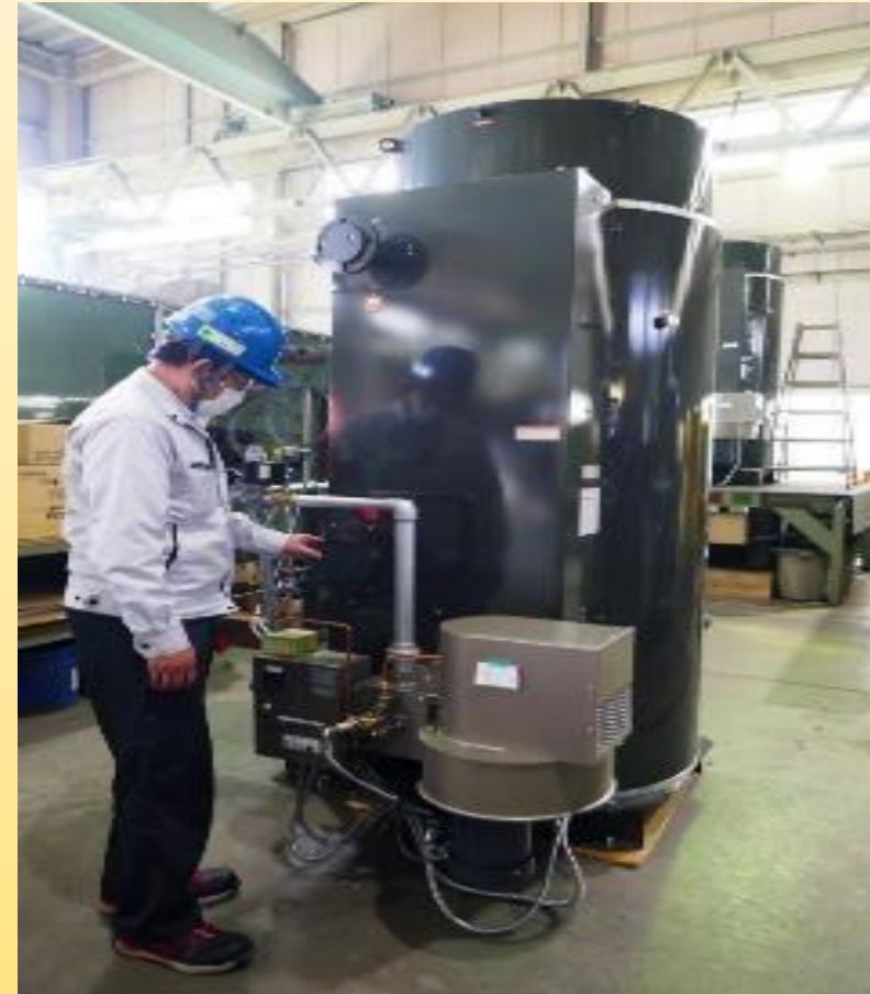
Gas boiler (372 kW) as an alternative to coal boiler
